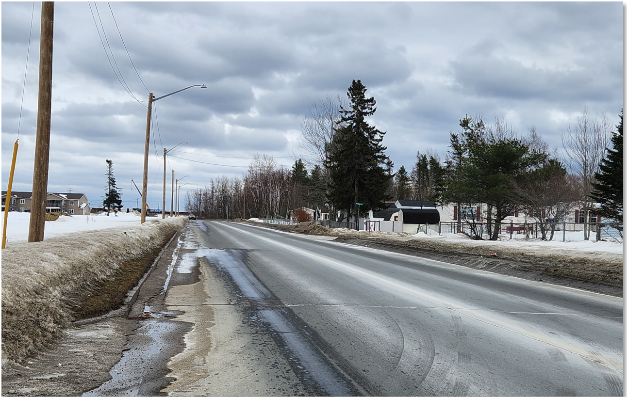
c. Photo 3: view of General Manson Way looking south.
