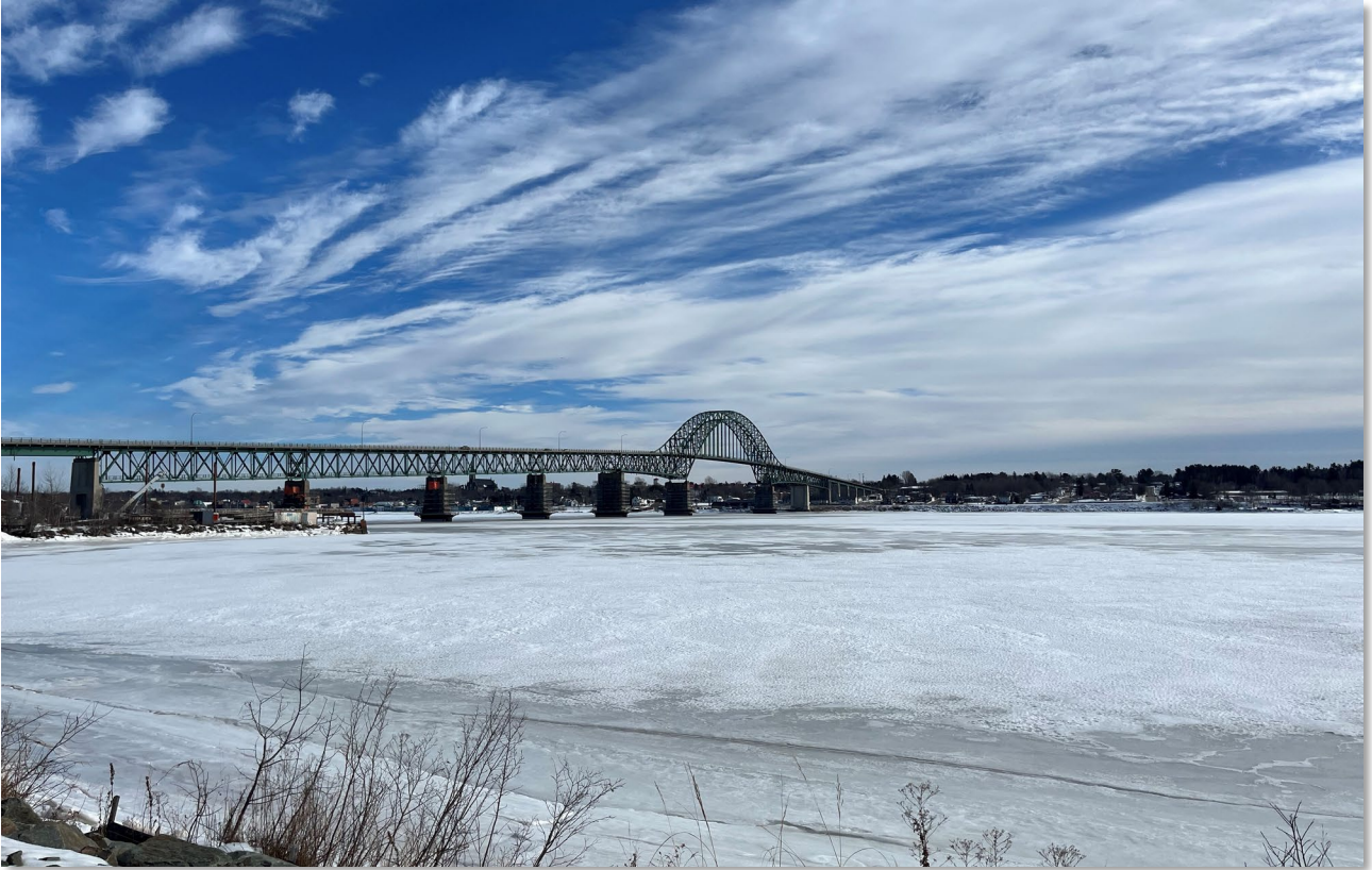
c. Photo 3: view of the Miramichi river, from the main entrance of the building
