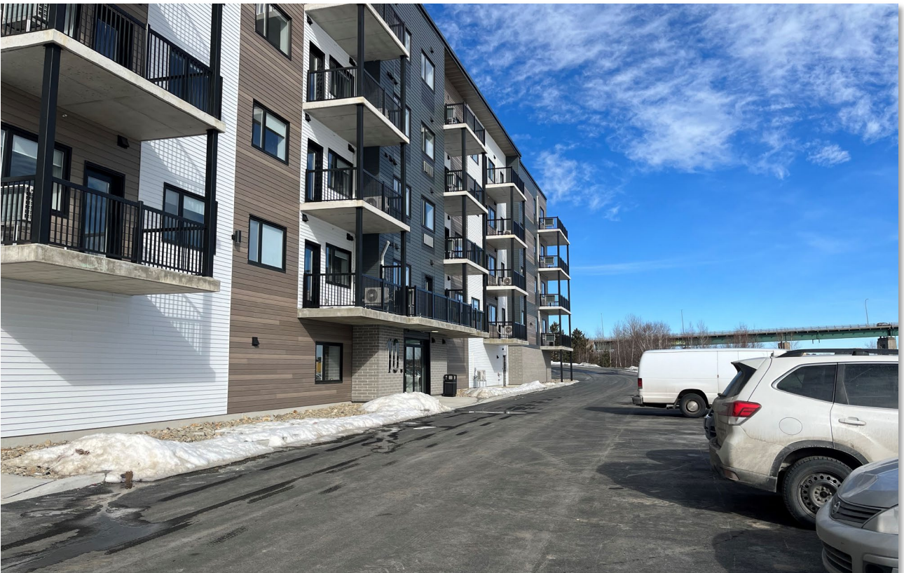
d. Photo 4: view of the existing building (phase 1), looking north-east.
